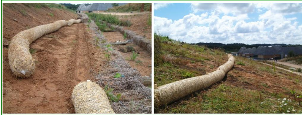
Straw Wattles help to stabilize slopes by shortening the slope length and there by slowing, spreading and filtering overland water flow. This helps to prevent sheet erosion as well as gully formation which occurs when water run-off flows uninterrupted down a slope. Straw Wattles retain sediment on the slope, therefore aiding re-vegetation and also preventing the sediment entering the water system.
